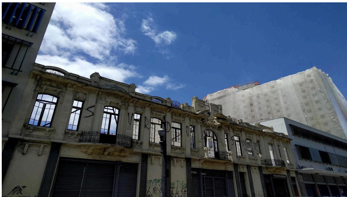
Fig 11: old building covered in graffiti next to a new building.
